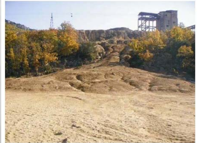
Mud overflowing from tailings pond extending to pond
